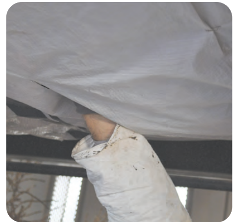
4. Cut access holes to ensure entire cavity will receive continuous and consistent insulation
