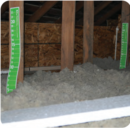
5. Depth rulers installed, 1 per 300 square feet
