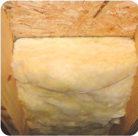
5. Batts are in good contact with subfloor
