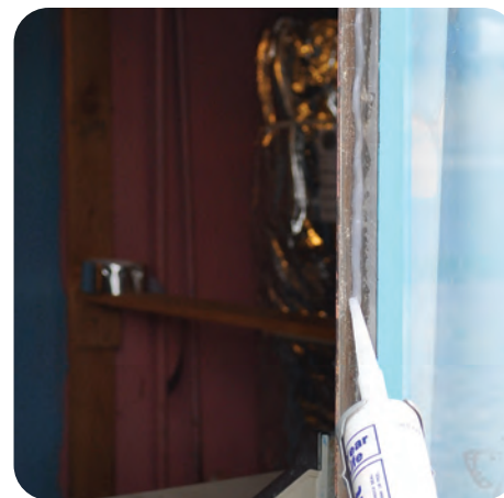
4. Run interior bead of caulk
