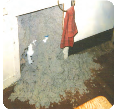
3. Ensure wall integrity is complete (no holes)
