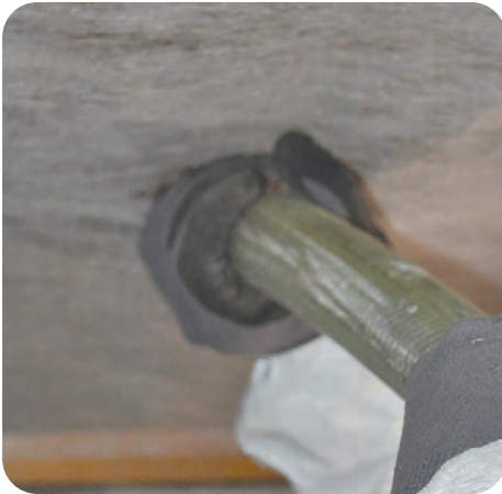
13. Loose fill netting to required density
