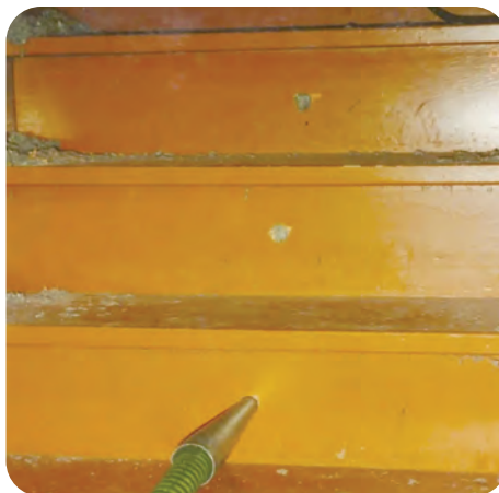
11. If backside of stairs is already sealed, blow insulation into cavity behind stairs
