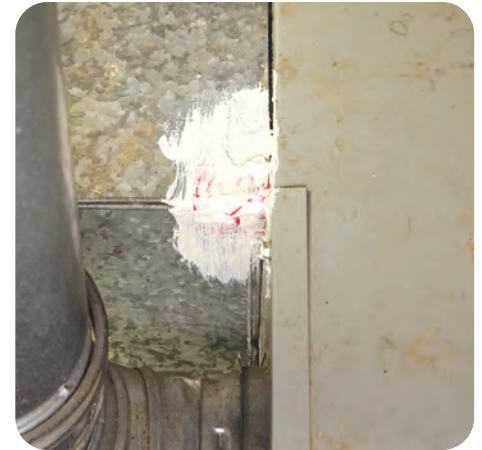
B-3. Apply mastic over the tape
